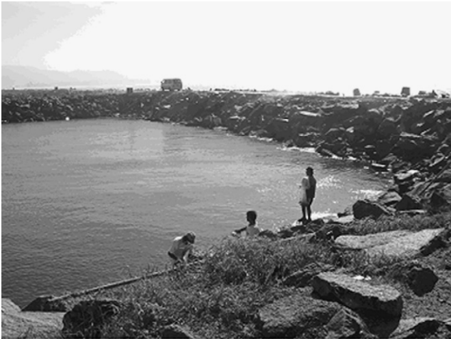
Fig. 5. The North Jetties. Photo by N. Peroni.
